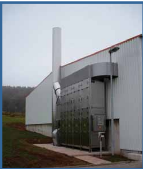
Sludge Storage - 10,000 cfm
