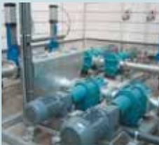
**In Waste Water Treatment Plants**, rags and stringy materials are often a problem for pumps, valves, instruments and controls and other downstream equipment. The Multicrusher with „Pull-In Function” macerates and reduces these troublemakers to unproblematic sizes.
