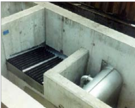
The Hydro-Jet Screen differs from conventional screening systems because the flow is passed across the surface of the screen rather than perpendicular to the screen.
