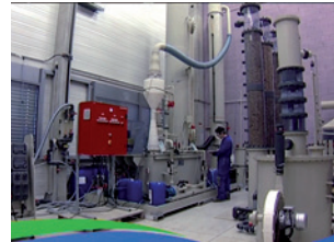
Pilot hall of more than 200 m 2
