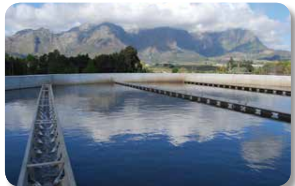
Treated effluent produced from an AquaNereda® reactor.
